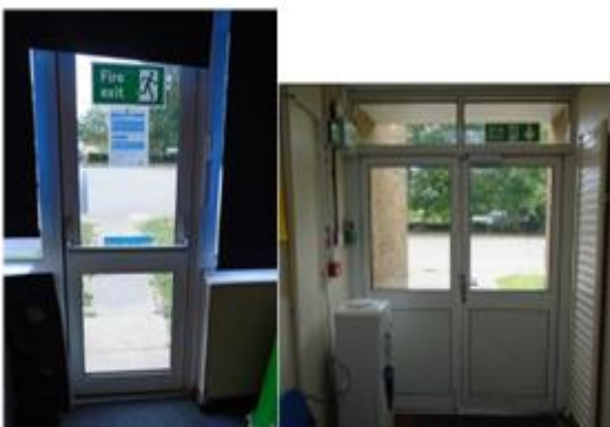
Doors to playground
